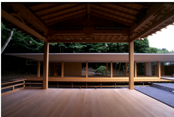
Noh Stage in the Forest, Miyagi Prefecture, Japan
